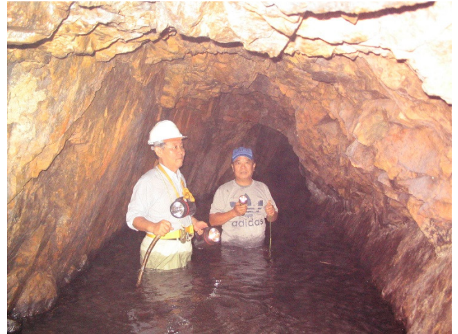
Fig.2 The first visit for the Silvermine Cave by Mr. Rocky Tan (The Executive Engineer from Meinhardt Consultant Ltd), and Mr. Teng Ka Hung (The Village Representatives) in the Lower Tunnel in 2007.
