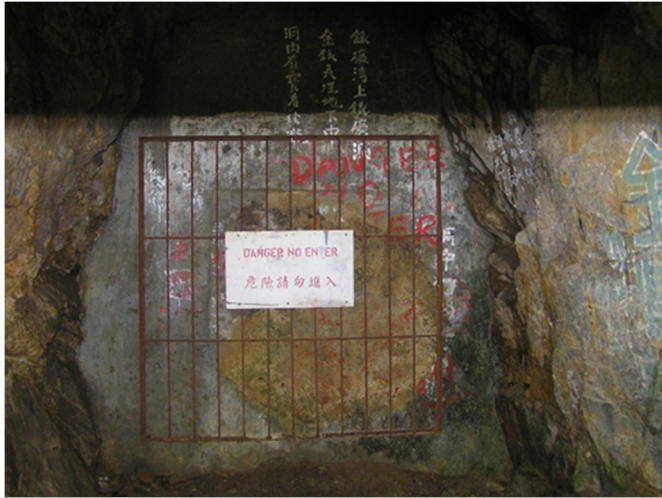
Fig.3 The Silvermine Cave was sealed by a concrete wall and steel barriers for safety reasons.
